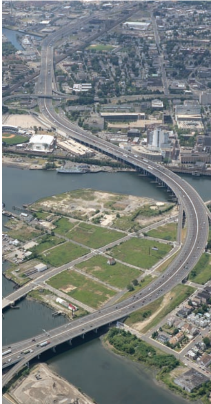
Connecticut is spending $200 million of the $1.6 billion it received on highway and bridge repair, including stretches of the state's major thruway, I-95.
